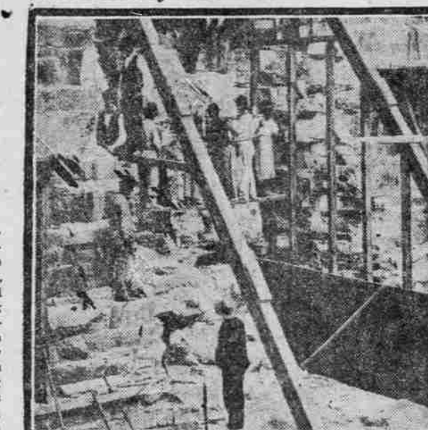
Digging out Rubble from Under the Base, to Replace With Concrete.
