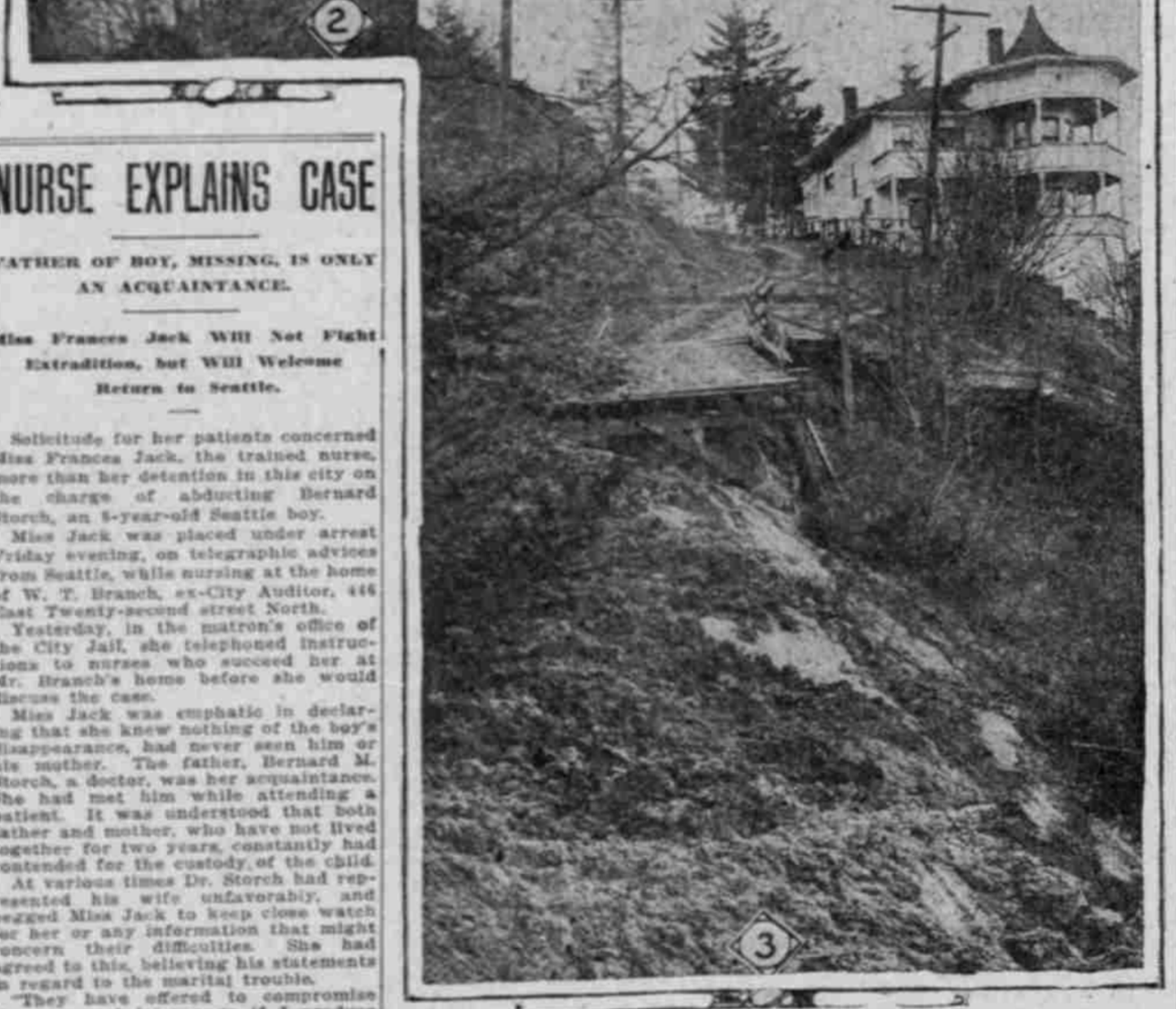
(1) Residence of Edward Holman, 440 Sixteenth street, showing slide to the East of the House; the Slide Did Great Damage and Threatened to Wreck the House; (2) Scene Where 30-Foot College-Street Bridge Was Hit by Slide and Carried Out. House Shown in the Picture Is Not Considered in Danger; (3) Home of Mrs. S. C. Long, Which Has Been Partly Wrecked by Slide to the Rear. Below the House is a Canyon. The House Has Settled Several Feet and the Roof Ridge Broken and the Walks Turn Out.
