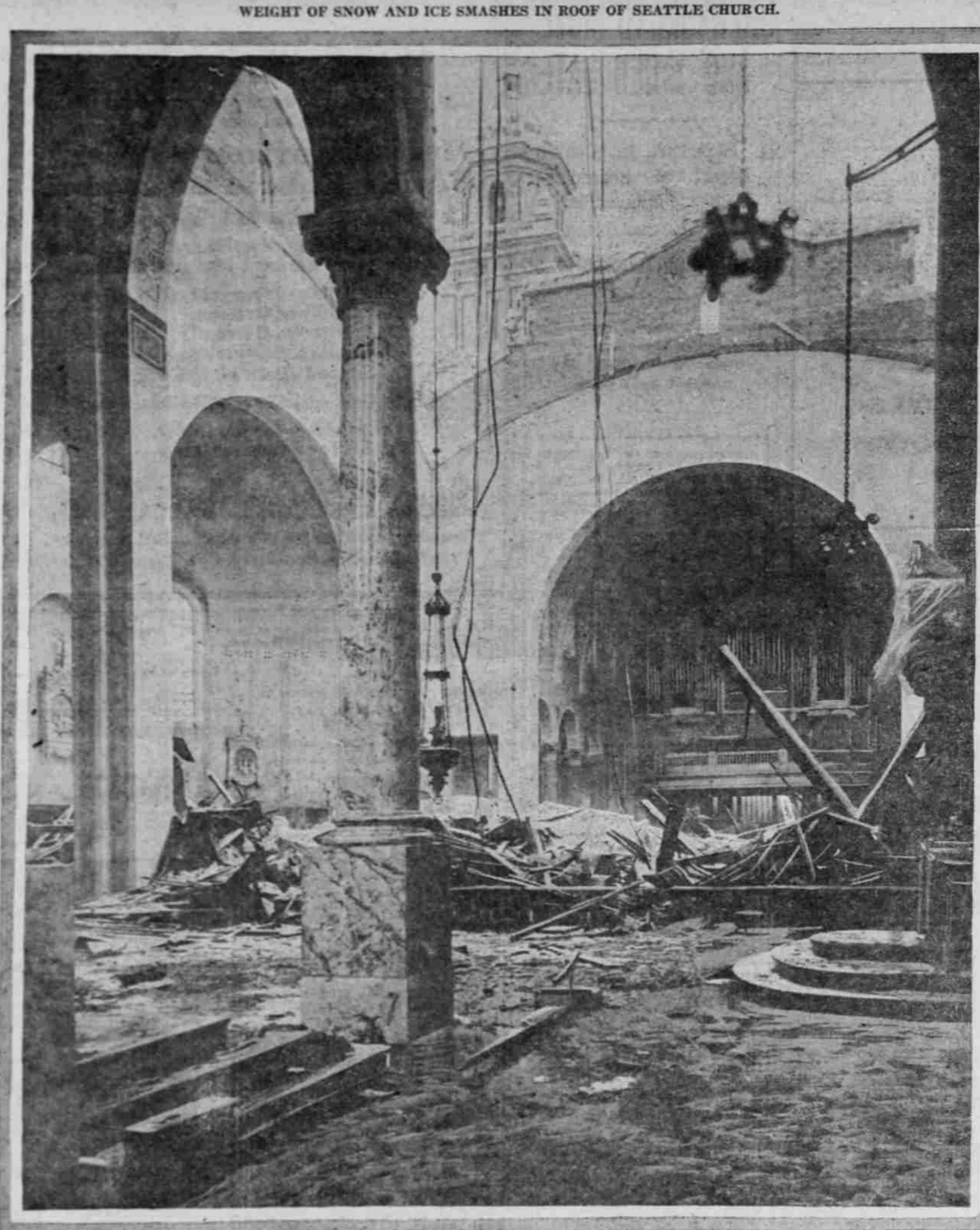
ST. JAMES' CATHEDRAL, SHOWING WRECKAGE FROM FALLEN ROOF AND ORGAN IN REAR.
