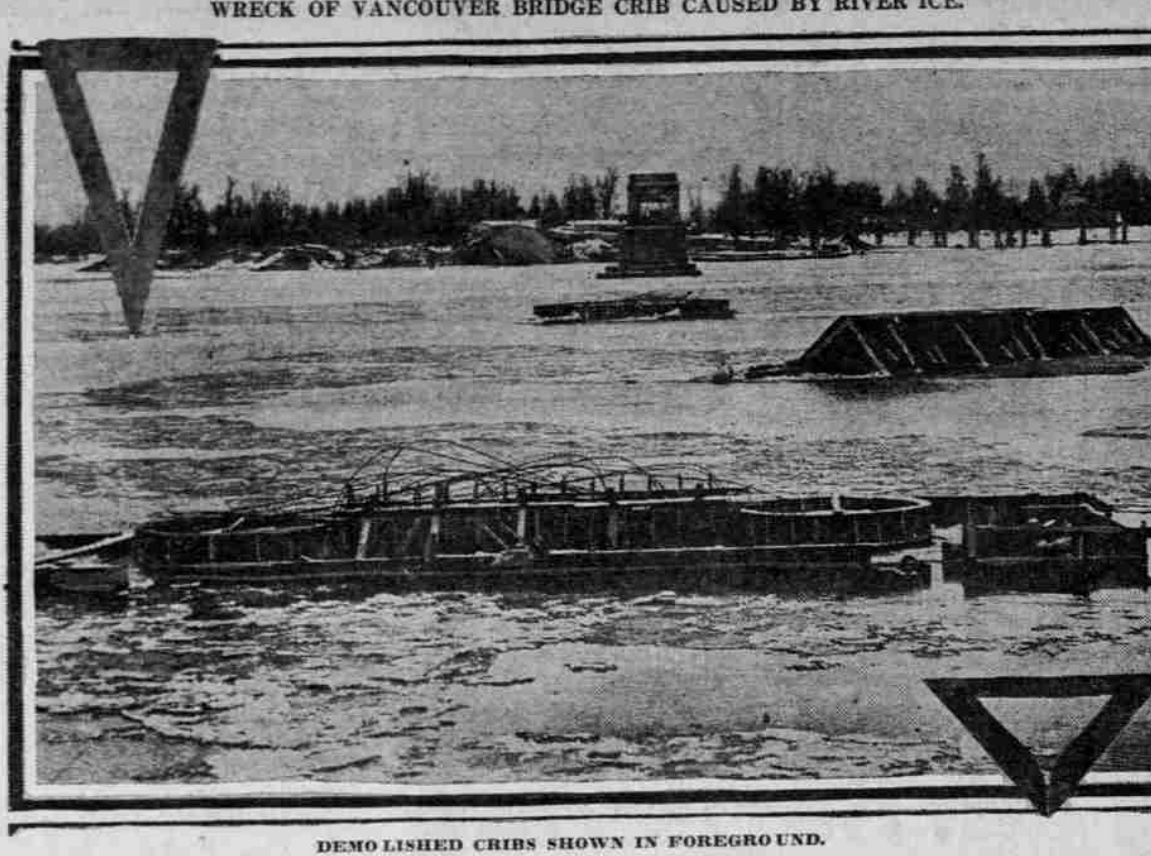
DEMOLISHED CRIBS SHOWN IN FOREGROUND.
