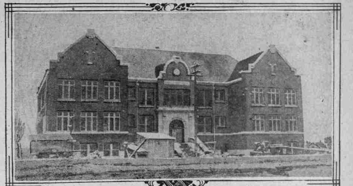
New Training School at Monmouth, Nearing Completion. —Illustration.
