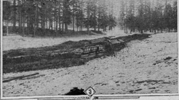
(1) Part of the Municipal Railroad Line Built for the Occasion. (2) One of the Two Busy "Dinky" Engines at Work With the Cars. (3) Engine in the Trench Ready to Move Loaded Cars. Engine is in Center of What Will Be Three-Acre Lake.
