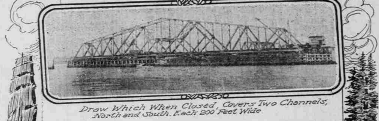
Draw Which When Closed, Covers Two Channels, North and South, Each 200 Feet Wide
