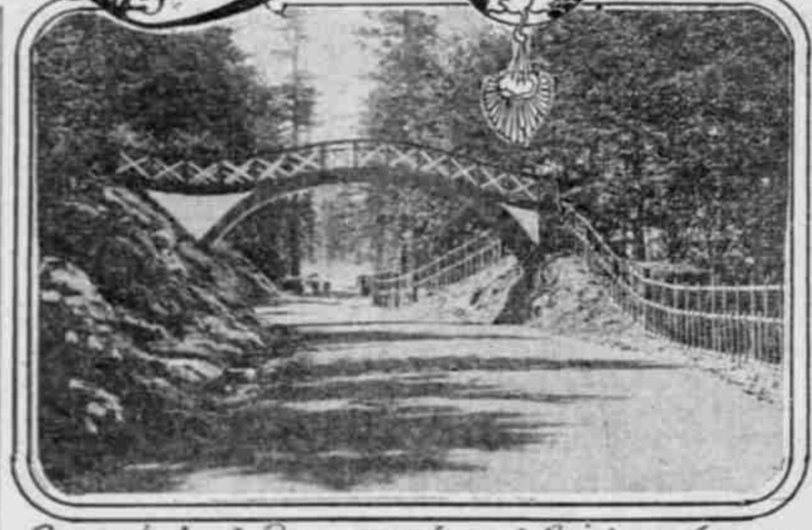
Completed Pavement and Bridge Across Highway.
