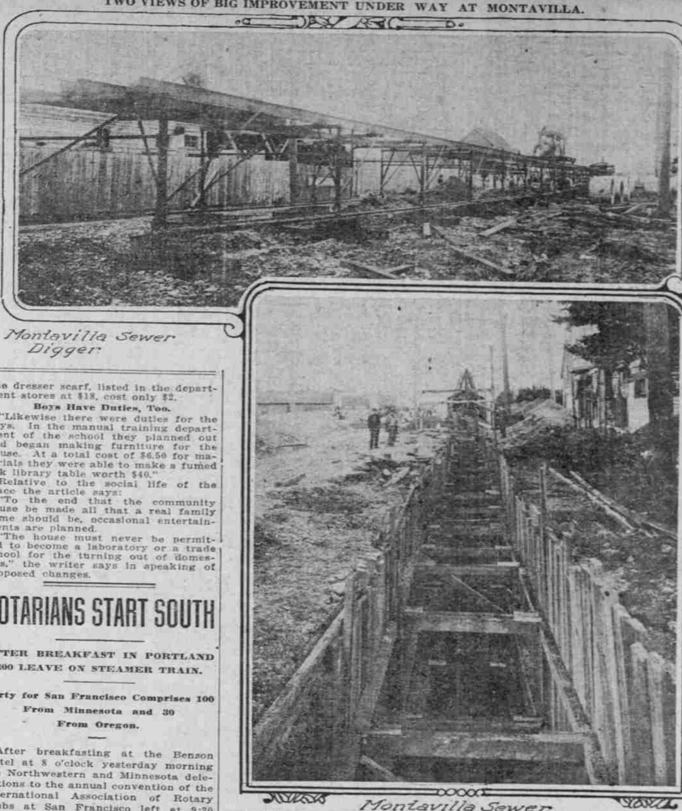
TWO VIEWS OF BIG IMPROVEMENT UNDER WAY AT MONTAVILLA.
