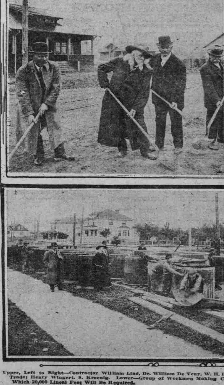
Upper, Left to Right—Contractor William Lind, Dr. William De Venz, W. H. Hamilton, President Montavilla Board of Trade; Henry Wingert, S. Kroenig. Lower—Group of Workmen Making Concrete Section of the Sewer Pipe, of Which 20,000 Lineal Feet Will Be Required.
