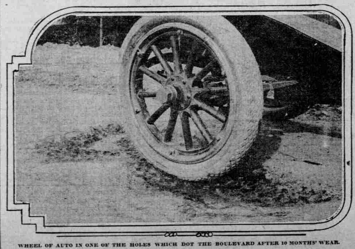
WHEEL OF AUTO IN ONE OF THE HOLES WHICH DOT THE BOULEVARD AFTER 10 MONTHS' WEAR.
