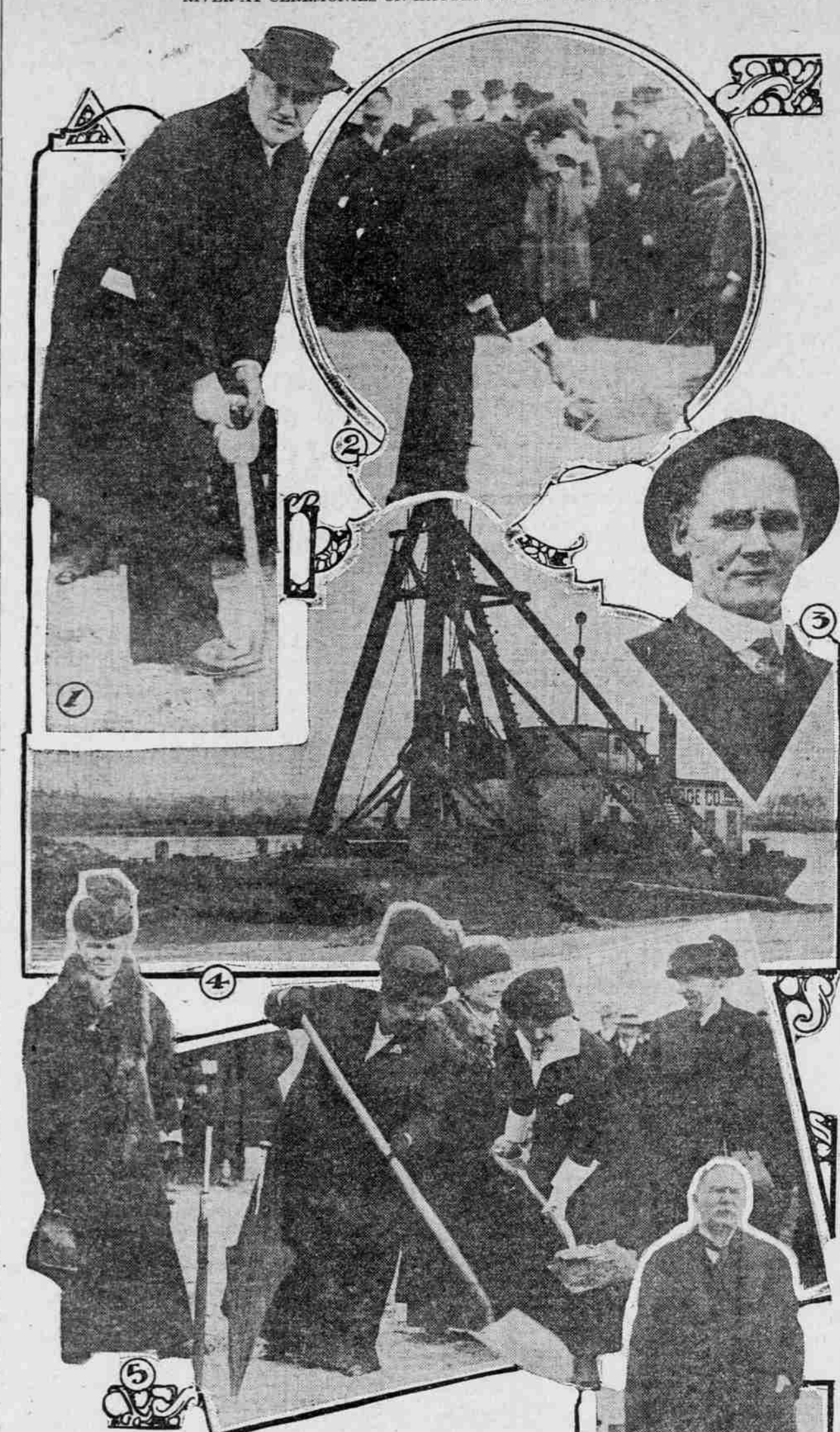
(1) County Commissioner Holman, (2) George L. Baker, (3) E. L. Beard, Master of Ceremonies; (4) Dredge Unloading Gravel for Bridge Work; (5) Women Take Hand in Breaking Ground for New Bridge; (6) W. P. Conaway, President Vancouver Commercial Club.
