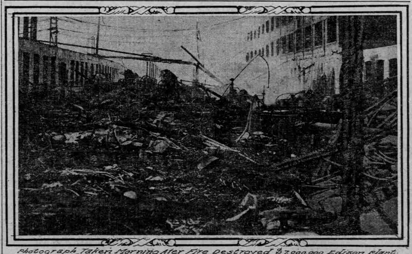
Photograph Taken Morning After Fire Destroyed $7,000,000 Edison Plant
