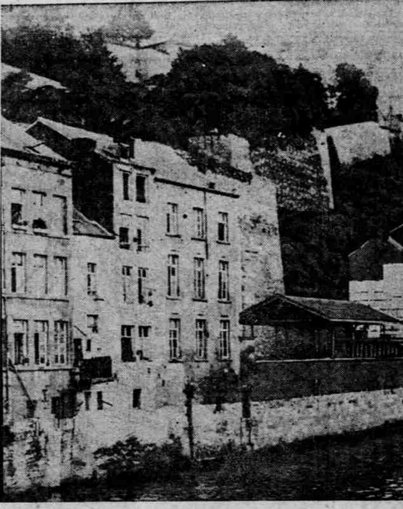
PHOTOGRAPH OF STRONGLY FORTIFIED CITY OF NAMUR, IN BELGIUM.
