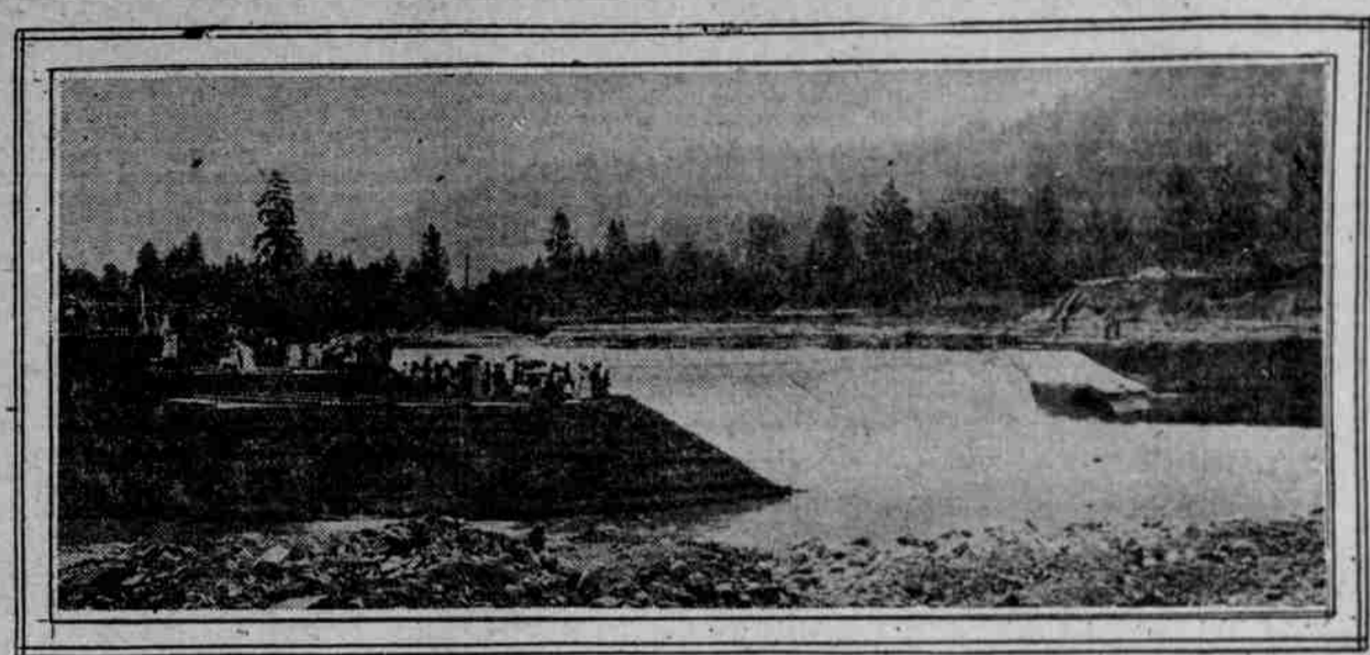
Dam Across Rogue River and Source of Intake
