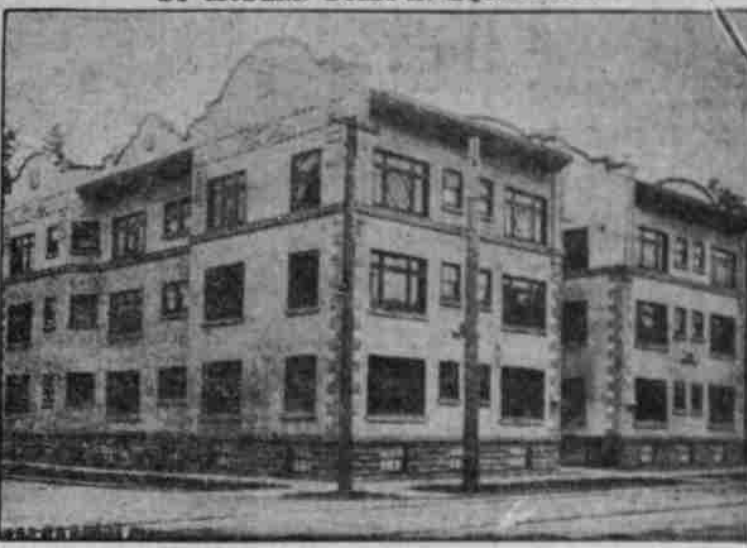
BARTLE COURT APARTMENTS. EUGENE, Or., June 27.—(Special.)—The new Bartle Court apartment-house in Eugene at a cost of $40,000, was thrown open to the public last week. It is the most modern equipped apartment-house in Eugene, with 24 two and three-room suites. The building is considered a model for its type of architecture. One particular feature is its built-in equipment. The kitchen in each apartment is a huge cabinet with even the ice chest an integral part. The beds not only fold up, but swing on hinges into a clothes closet.
