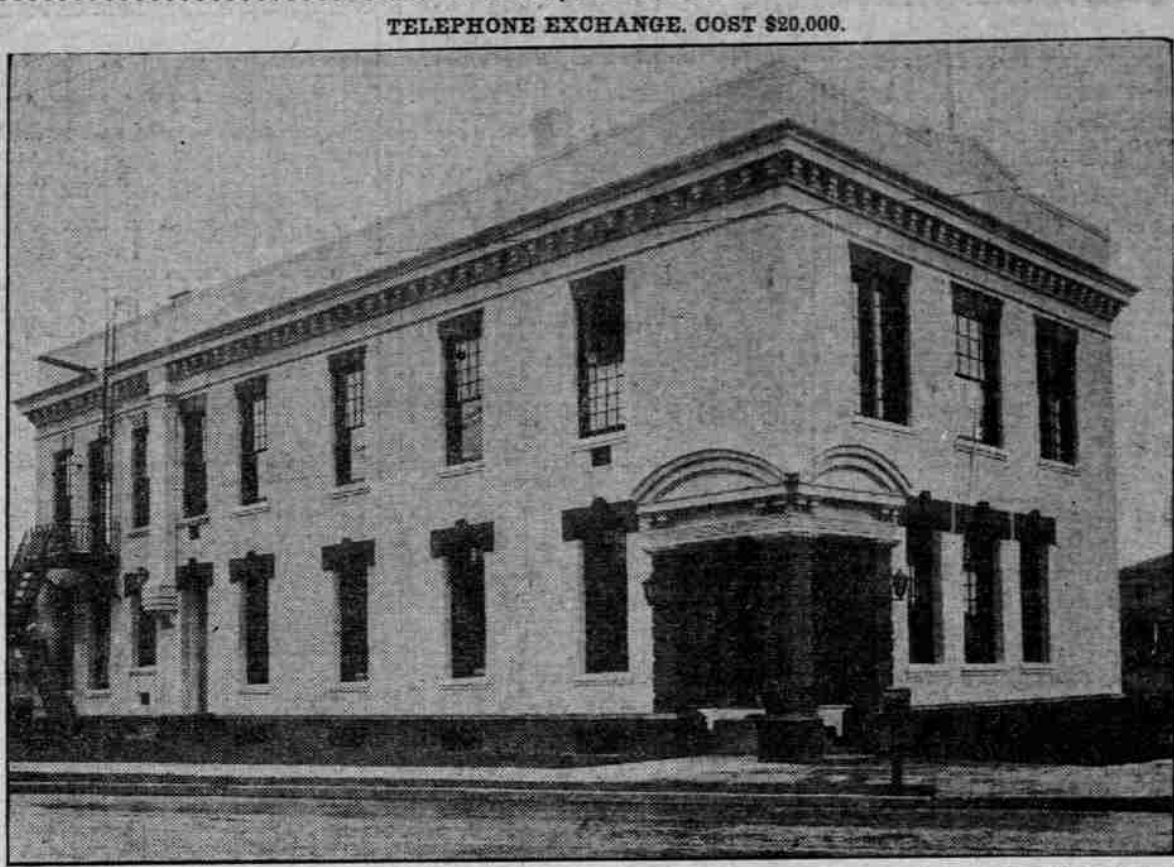
MOUNT TABOR EXCHANGE OF THE PACIFIC TELEPHONE & TELEGRAPH COMPANY AT EAST FIFTY-FIFTH AND BELMONT STREETS. The Pacific Telephone & Telegraph Company has remodeled and enlarged its Mount Tabor exchange, at the southeast corner of Belmont and East Fifty-fifth streets. The structure has been generally improved at an expense of about $20,000.
