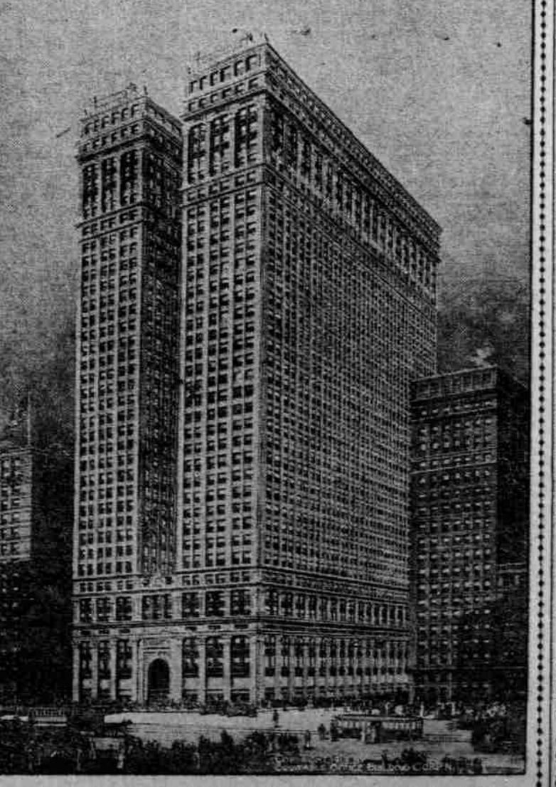
EQUITABLE BUILDING, UNDER CONSTRUCTION IN NEW YORK.
