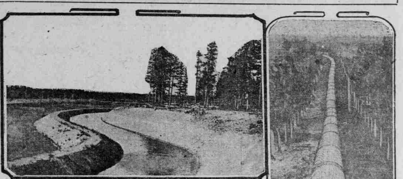
The Deschutes Land Co. Main Canal.
