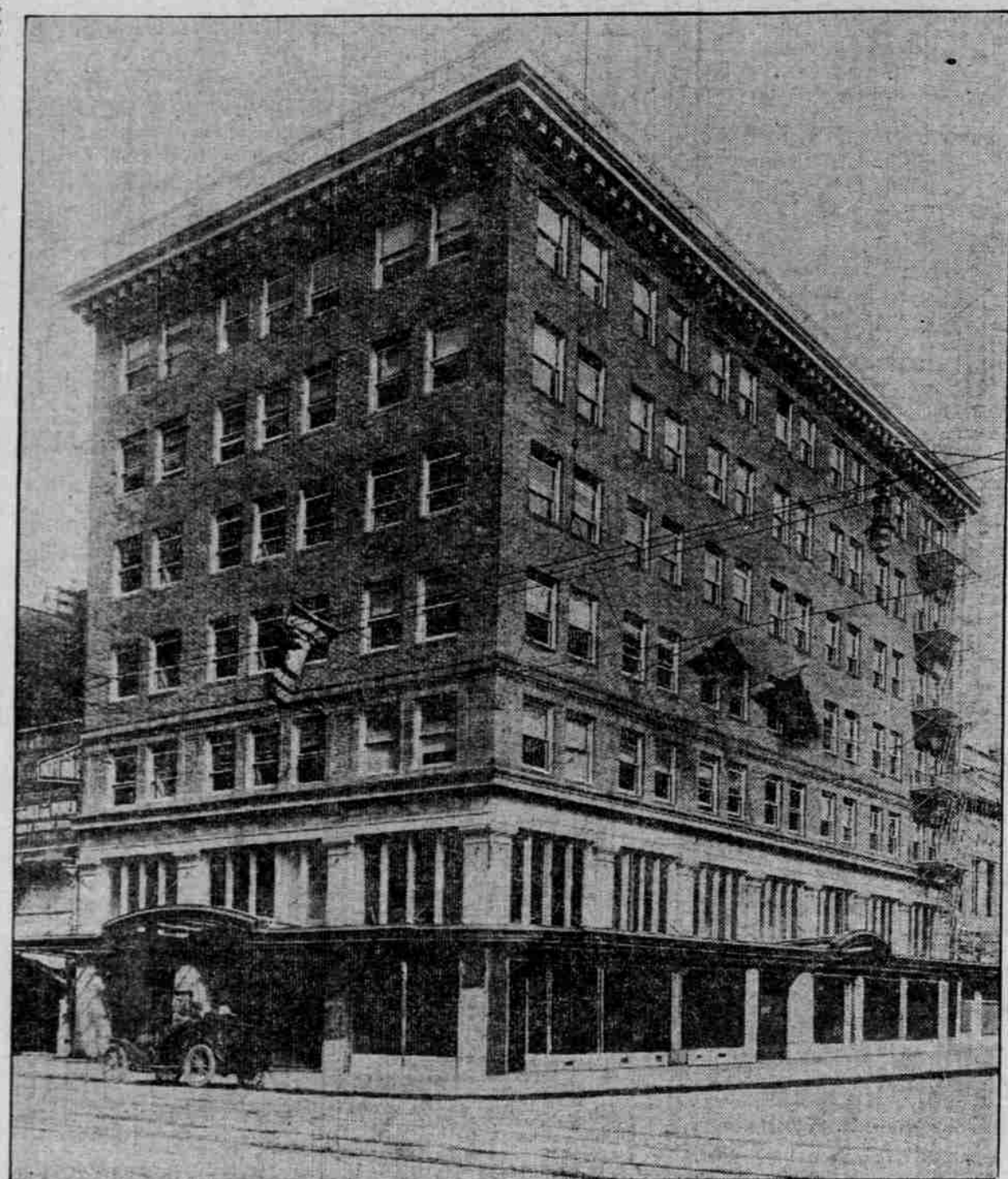
TWO STORIES MAY BE ADDED TO STRUCTURE THAT COST $105,000.
