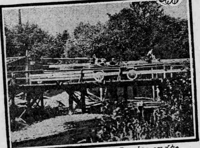
Crossing a Condemned Bridge on the Pacific Highway.
