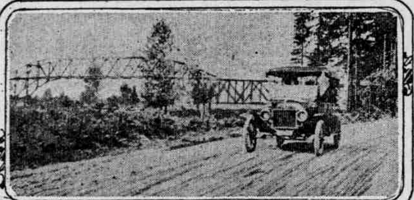
The New Steel Bridge at Woodland, Wash., Pacific Highway.
