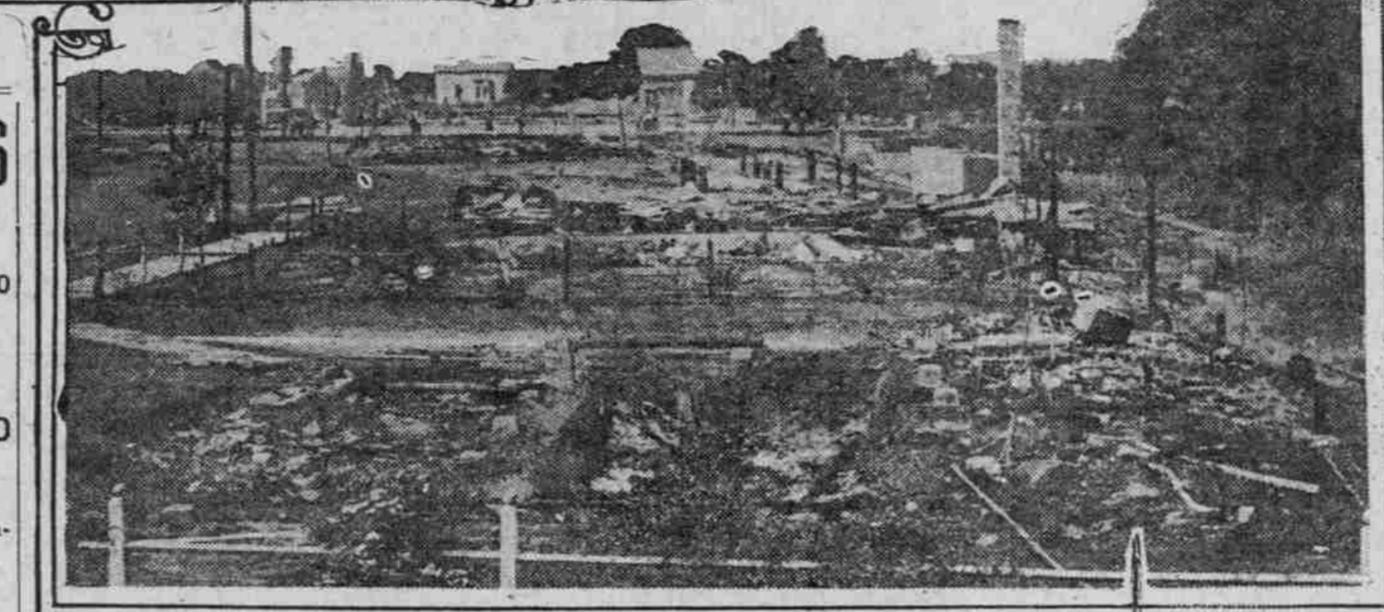
Birdseye View of Ruined Section, Looking West
