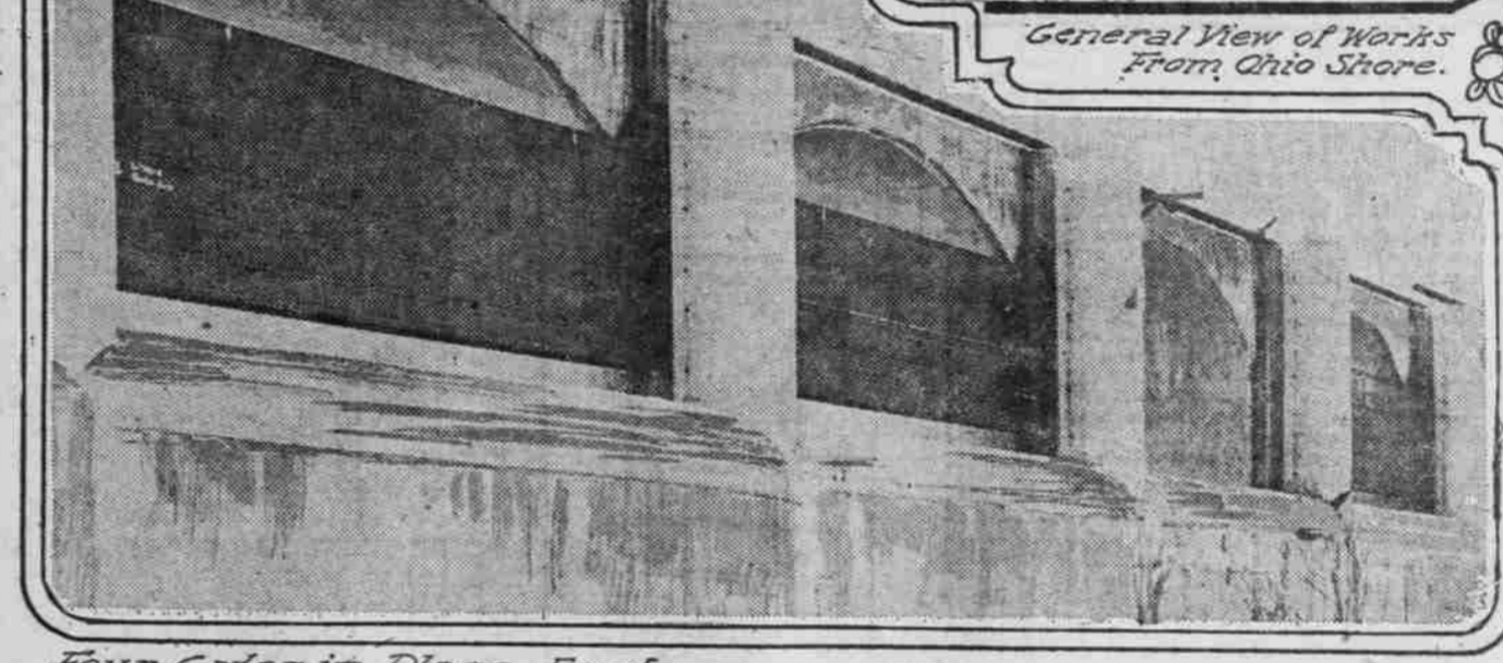
Four Gates in Place, East End of Dam.
