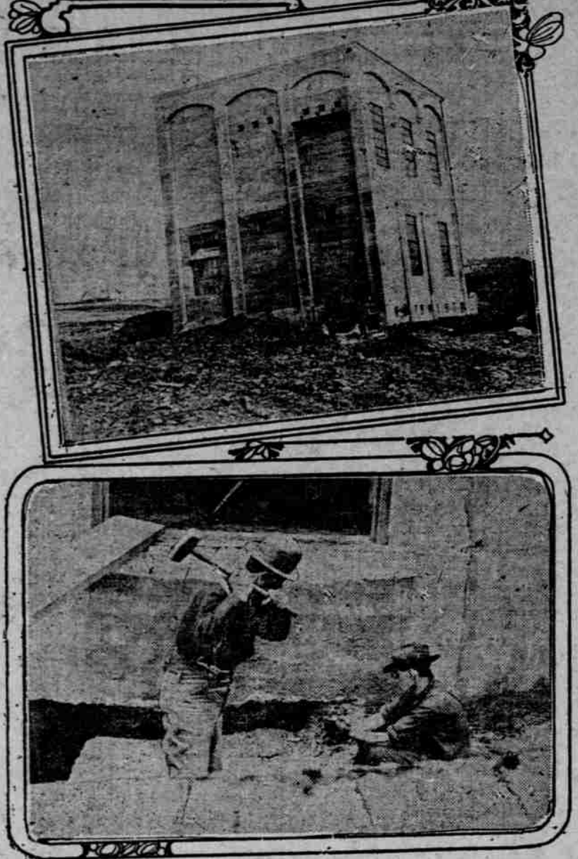
ABOVE, CONCRETE POWER STATION WHICH IS BEING MOVED—BELOW, WORKMEN ATTACKING WALL.
