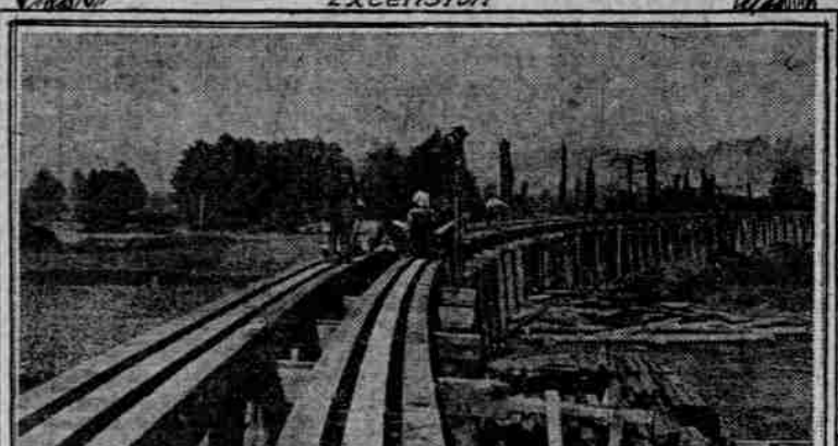
1500 feet of Trestle Being Built Over River
