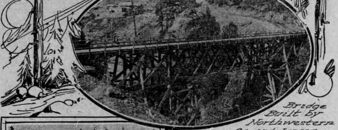
Bridge Built by Northwestern Co. and Lower Camp.
