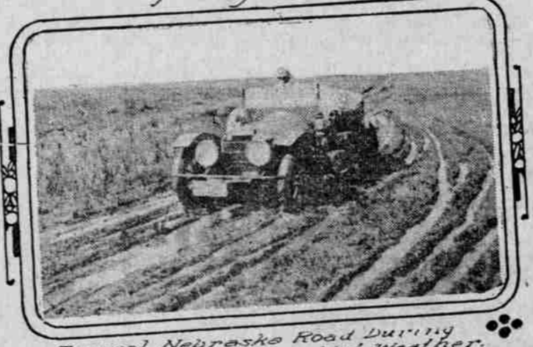
Typical Nebraska Road During Wet Weather.
