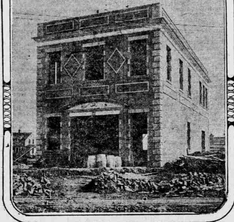
New Fire House Rose City Park
