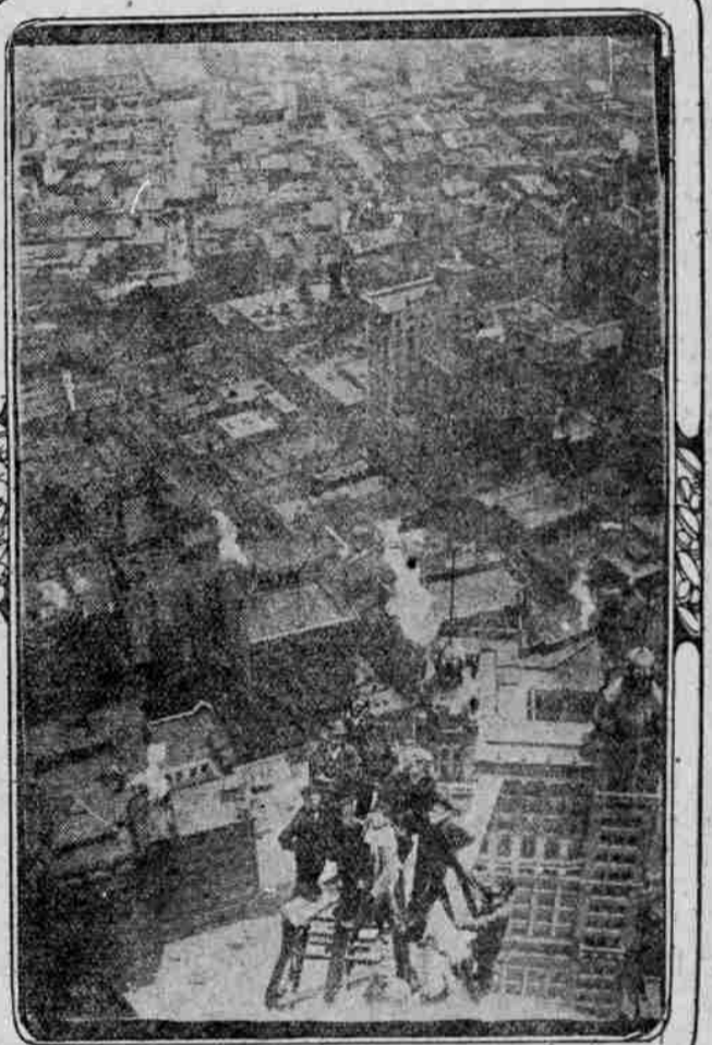
Workers on Top of Woolworth Bldg., N.Y.
