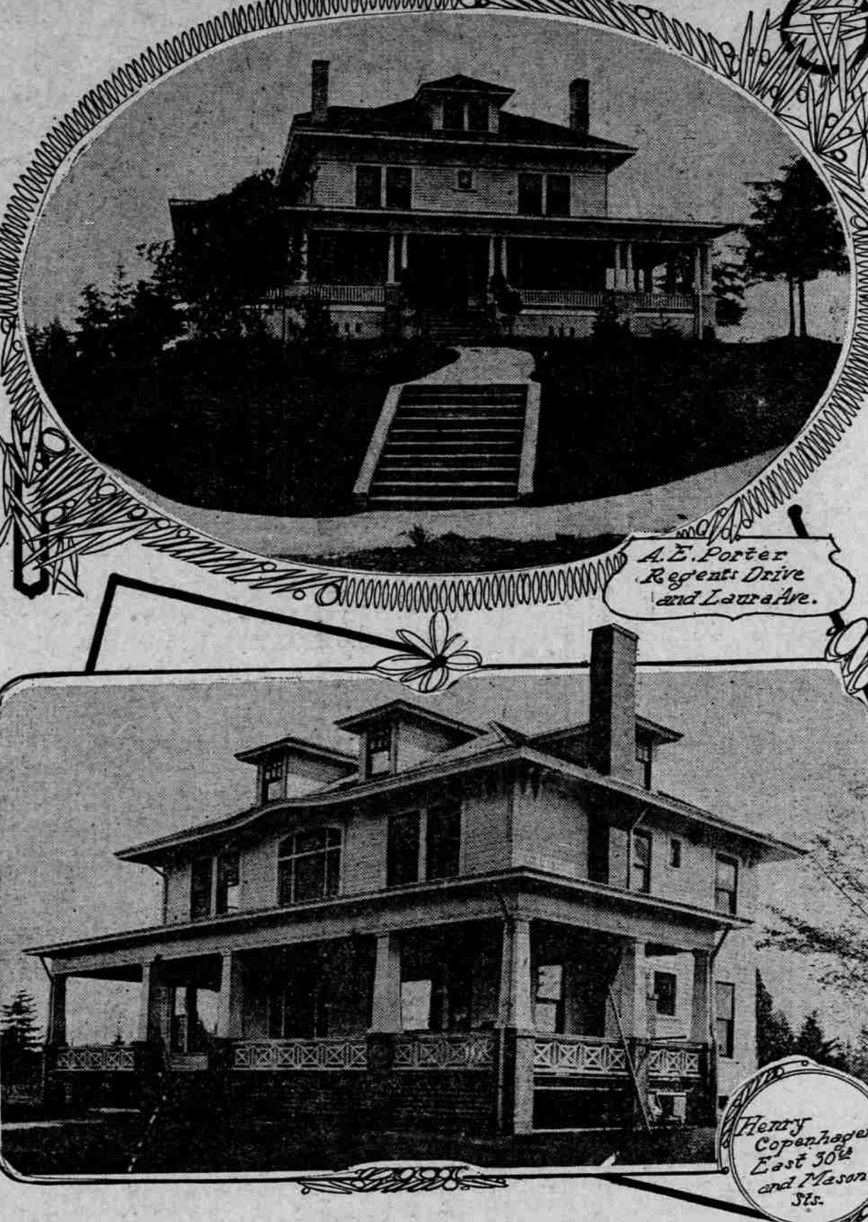
Among the Attractive Homes Erected in Alameda Park Are Those of A. E. Porter, at Regent's Drive and Laura Avenue, and Henry Copenhagen, at East 30th and Mason Streets.
