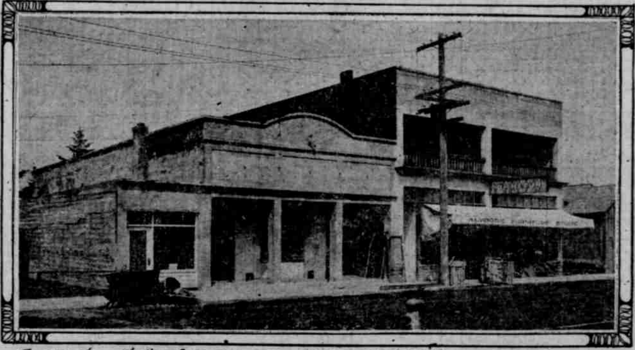
Concrete Blgd. of H.E. Brous, Kern Park Station, 46th Avenue, and East 67th St.
