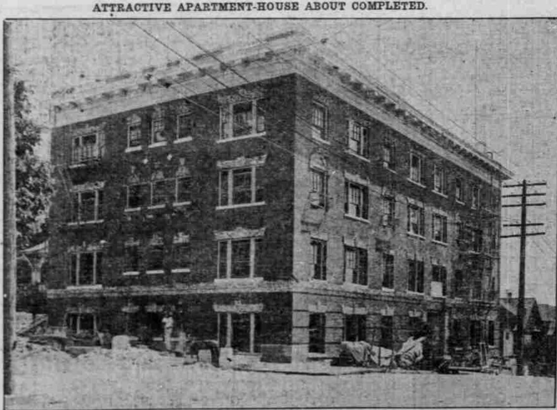
EAST SIDE STRUCTURE BUILT FOR M. OLSEN AT COST OF $50,000.
