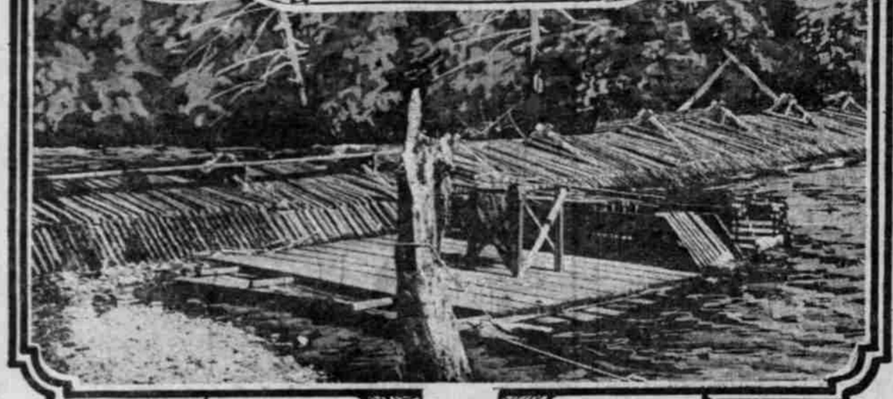
Rack And Upstream Trap On Salmon River.
