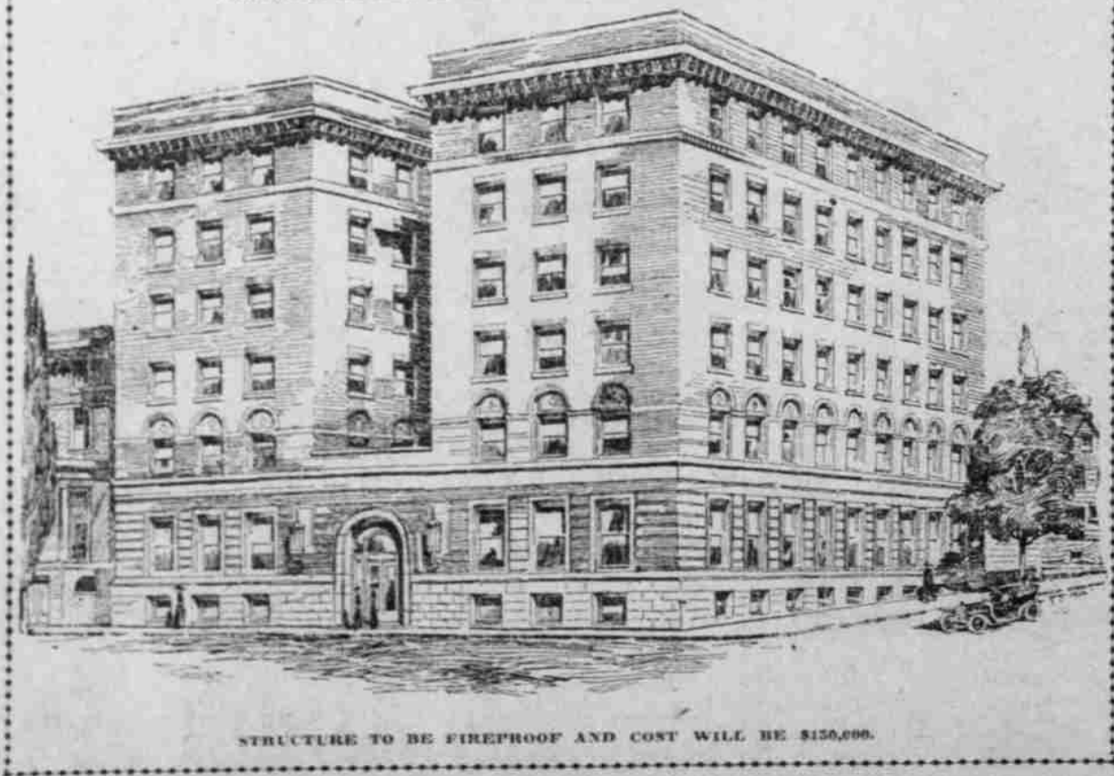
STRUCTURE TO BE FIREPROOF AND COST WILL BE $150,000.
