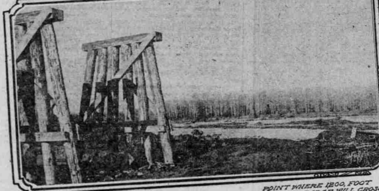
POINT WHERE 1200 FOOT STEEL BRIDGE WILL CROSS SANTIAM RIVER.
