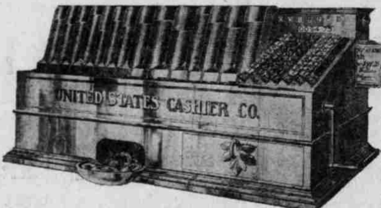
AUTOMATIC BANK CASHIER A change-making, listing, adding, check-cancelling and coin-paying machine, designed for banks and payrolls. Pays any amount, 1c to $200.00. Permanently lists, visibly registers, prints amount on check and totals each transaction.
