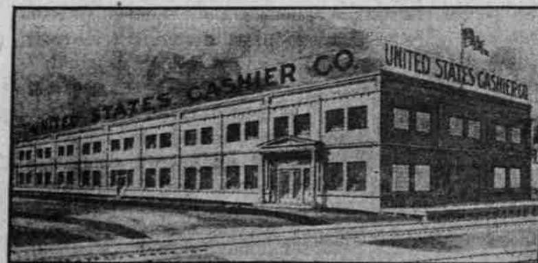
THE NEW, MODERN FACTORY View of the large new concrete factory of the U. S. Cashier Co. at Kenton. The installing of special machinery is now going on.
