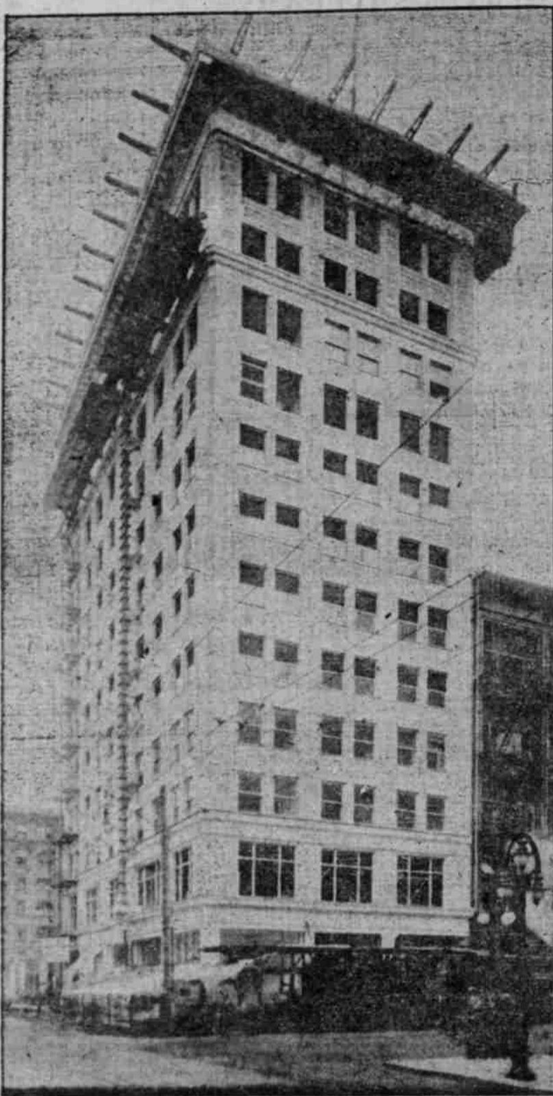
EXTERIOR OF TWELVE-STORY STRUCTURE COMPLETED.
