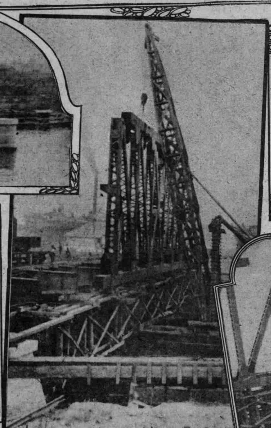
PLACING HEAVY GIRDERS
