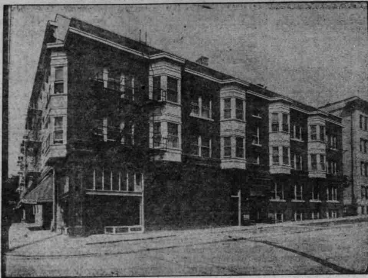
BUILDING SHOWS HOW SMALL TRACT CAN BE MADE INTO DIVIDEND PAYER. Work on the new hotel building on Washington street and Trinity place, built by Mrs. Nettie A. Garland, has been completed and is ready for occupancy. The building is three stories high and 30 by 100 feet in size and equipped with all modern hotel conveniences. The exterior is of tapestry clinker brick. There are 30 rooms, each with hot and cold water. Most of the rooms are fitted with bath. The building was erected by John Alemeiter. The plans were drawn by Williams & Roanbeck, architects. On the lower floor are store rooms, and in the basement is a place for a barber shop and other hotel accessories. Mrs. Garland holds the new building as a sample of what can be done on a small piece of Portland property. "People are complaining about property being so high," says Mrs. Garland. "The trouble is they do not know how to improve property. This lot, which is 20 by 100 feet in size, was purchased six years ago, and now, with the improvements, which are really not large, pays interest on $50,000." A five years' lease has been taken on the building by Phil Gevarts.
