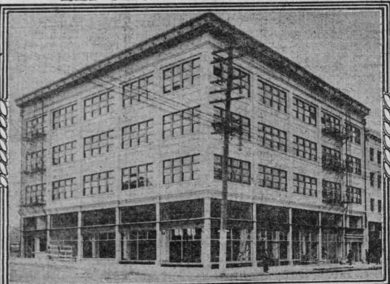
J. R. CARTWRIGHT BLDG. GRAND AVENUE AND EAST OAK STREET.
