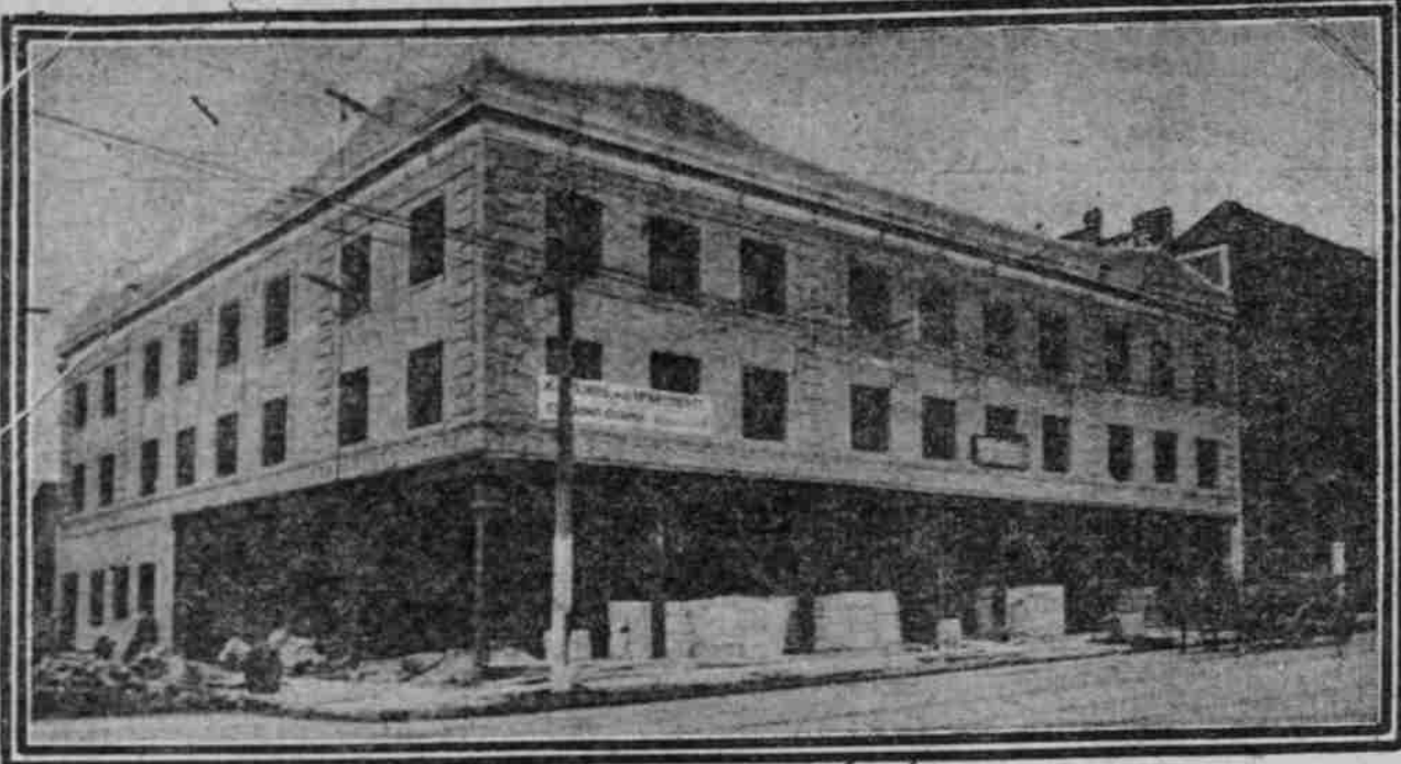
STANLEY BOISE & SMITH BLDG., EAST 6TH STREET AND HAWTHORNE AVENUE.
