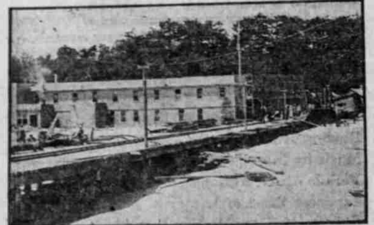
CONSTRUCTION SCENE AT BAYOCEAN.
