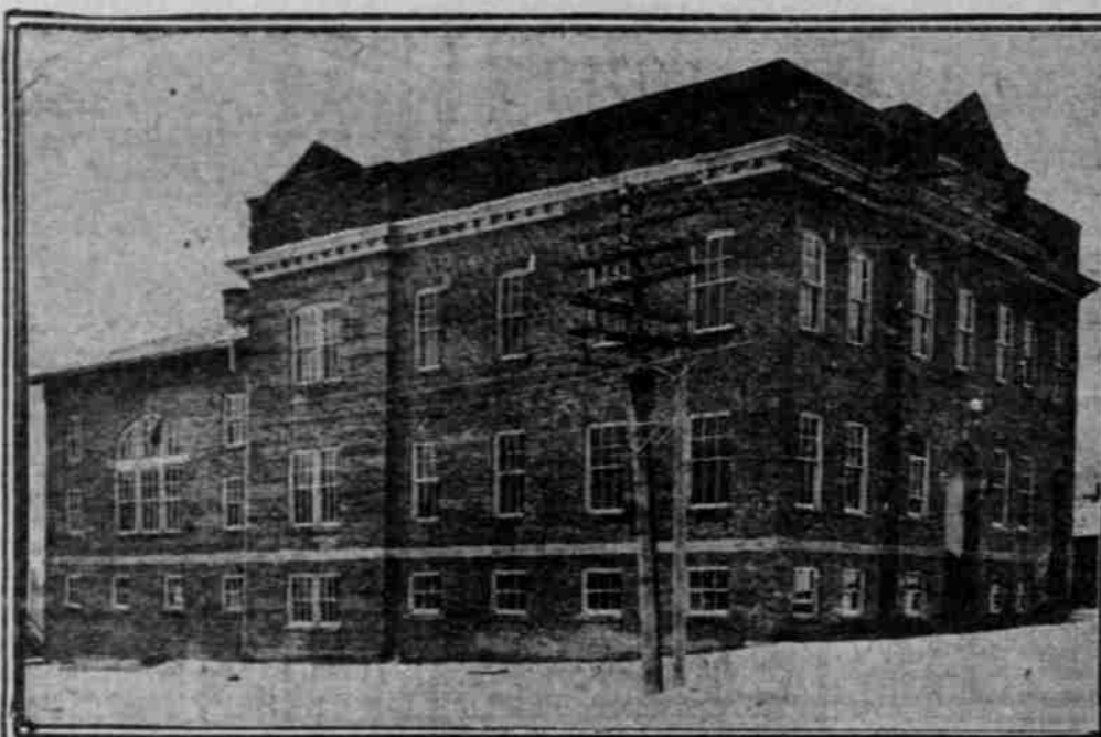
INDUSTRIAL Y.M.C.A. BUILDING, KELLOGG, IDAHO.
