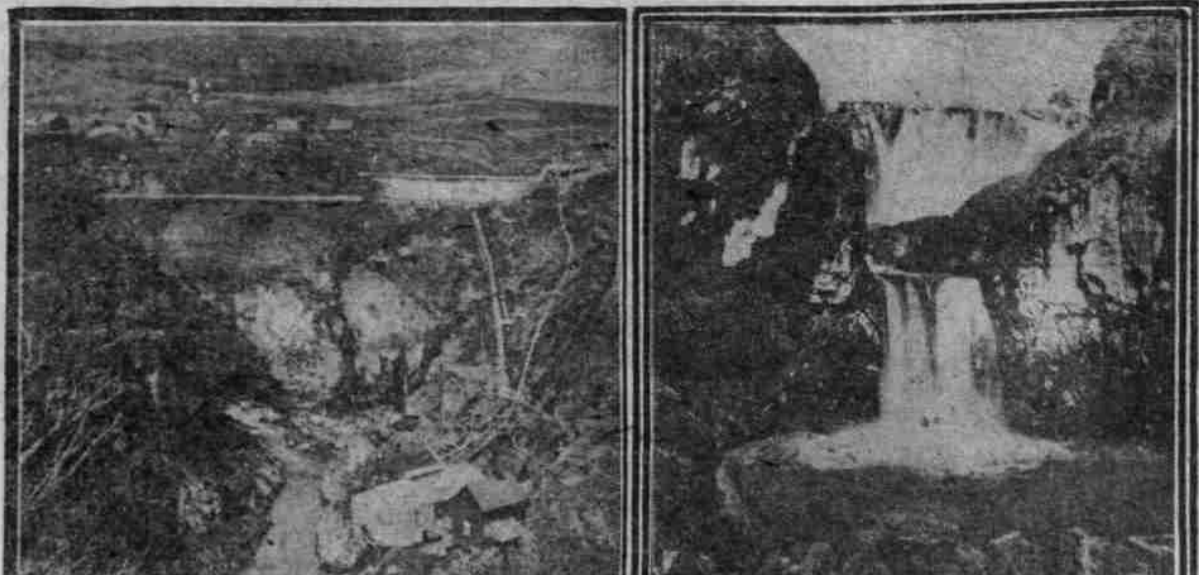
POWER HOUSE DAM AND PIPE LINE, WHITE RIVER FALLS
