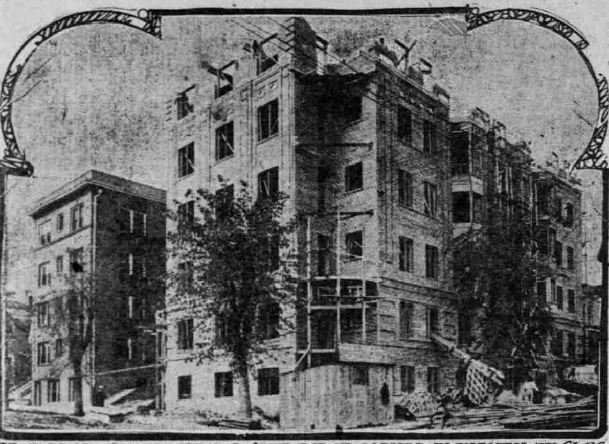
CLAYPOOL APARTMENTS, SOUTHWEST CORNER ELEVENTH AND CLAY.
