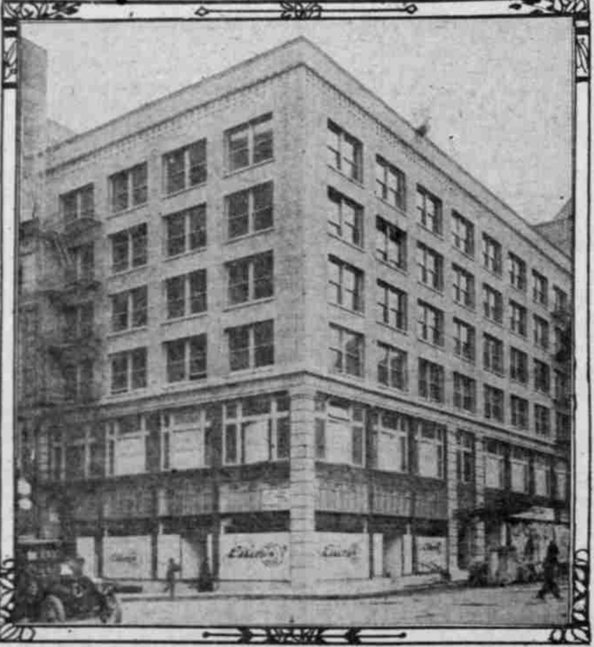
HARGLY-TICHTNER BUILDING, SEVENTH & ALDER.
