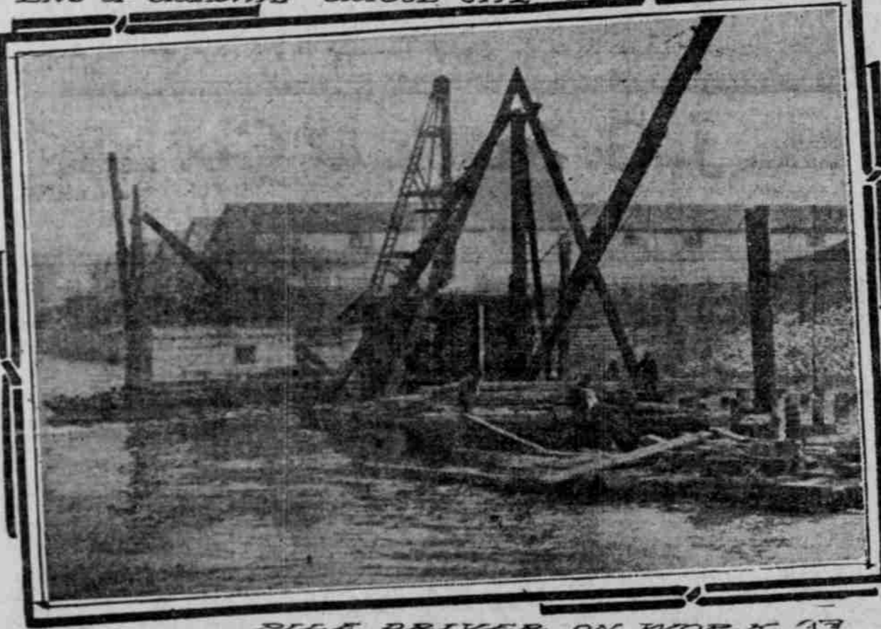
PILE DRIVER ON WORK AT EAST END OF BROADWAY BRIDGE
