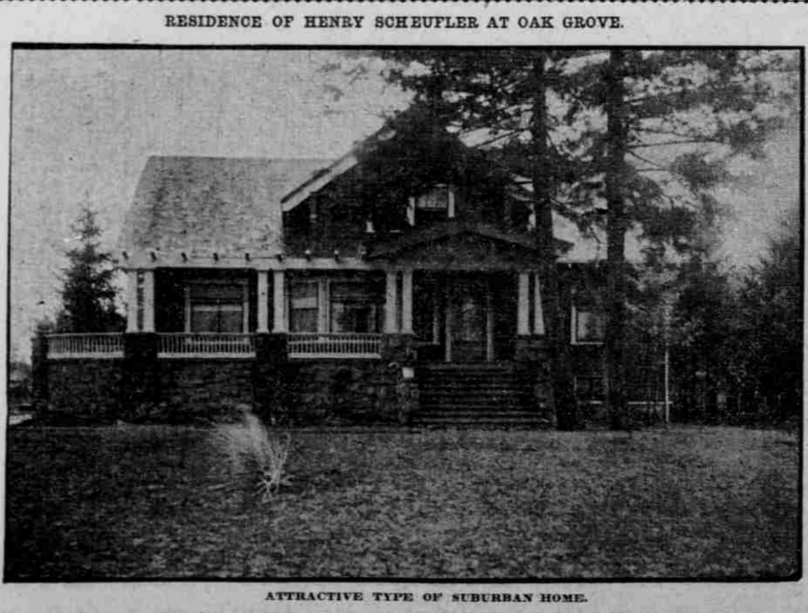
RESIDENCE OF HENRY SCHEUPLER AT OAK GROVE. ATTRACTIVE TYPE OF SUBURBAN HOME.
