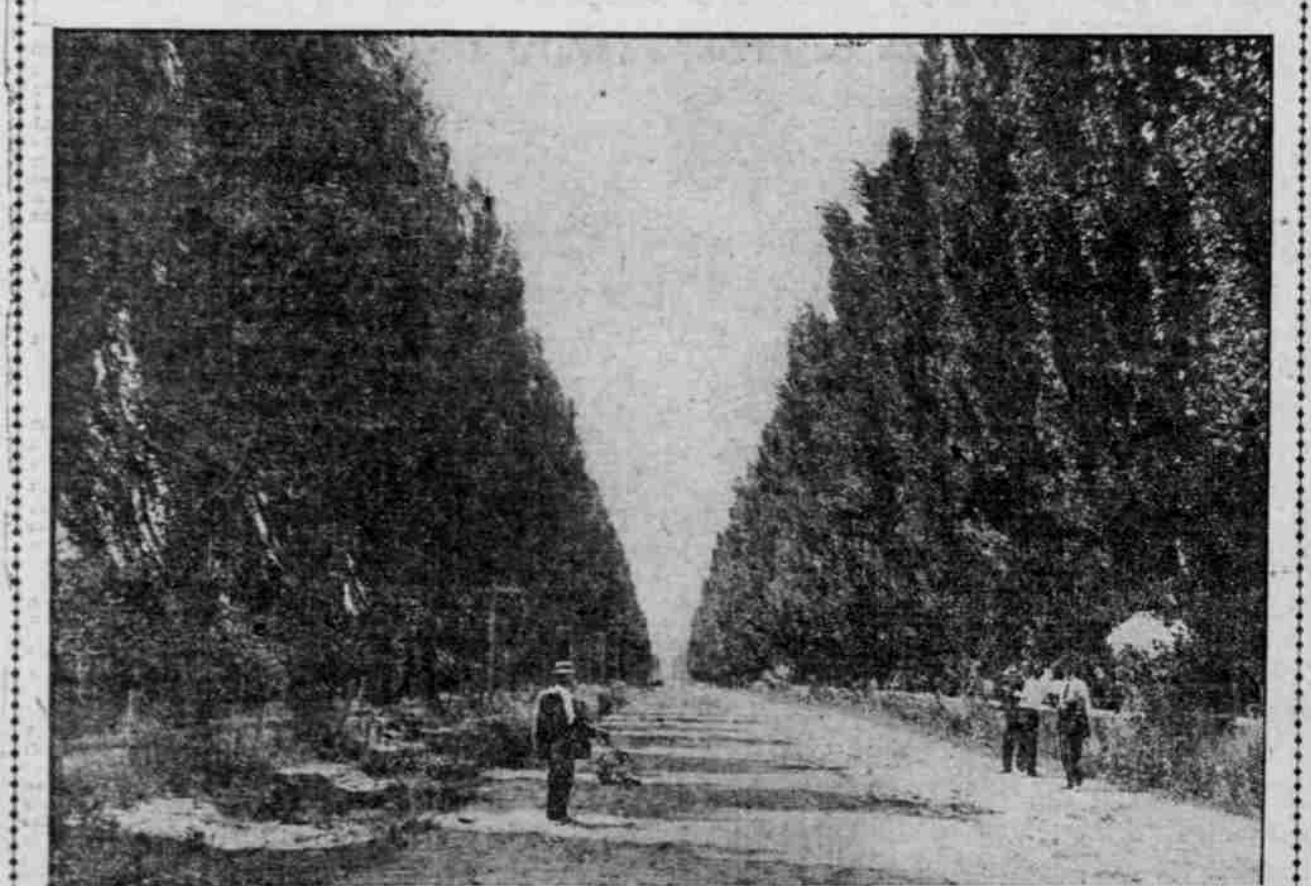
SIX-MILE AUTOMOBILE BOULEVARD SOUTH OF ONTARIO.
