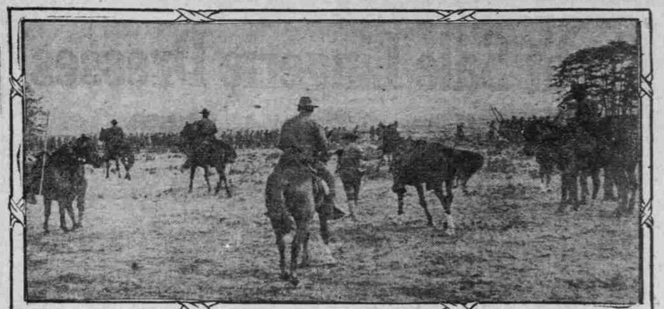
SIGNAL CORPS GETTING READY TO LAY FIELD TELEPHONE LINE.
