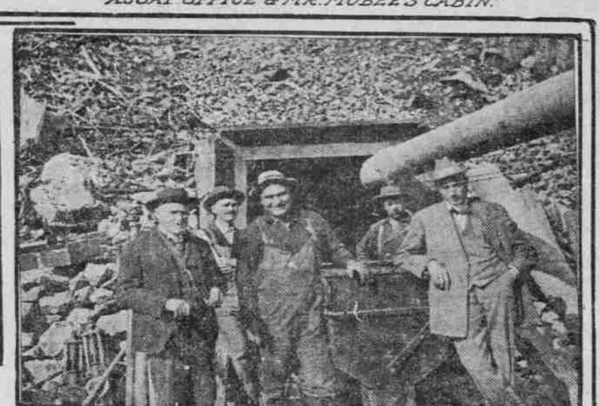
PORTAL OF SOUTH TUNNEL.
