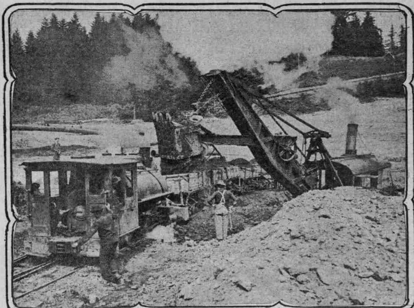
STEAM SHOVEL LOADING DIRT TRAIN IN NEW CITY RESERVOIR NO. 6.
